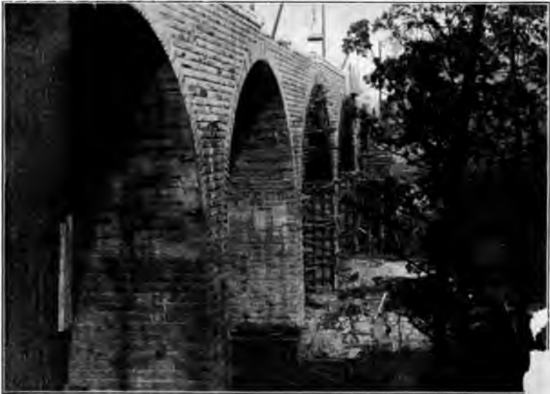
NEW BRANDYWINE VIADUCT OF THE BALTIMORE & OHIO, AT WILMINGTON, DEL.
